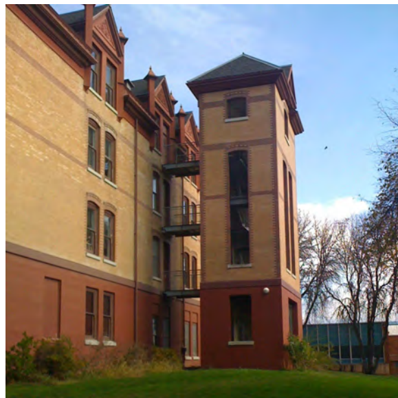
New construction on the Oregon State University campus provides additional egress to the historic building.
